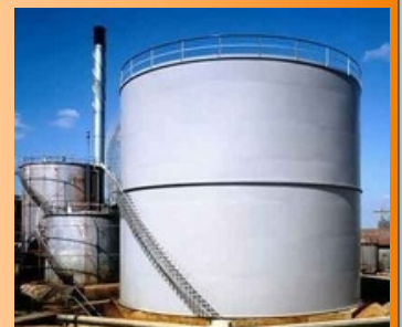
Storage Vessels (For General Purpose- All Industry)
